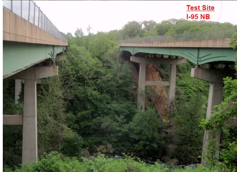
Figure 9 - I-95 NB Bridge over Patuxent River
