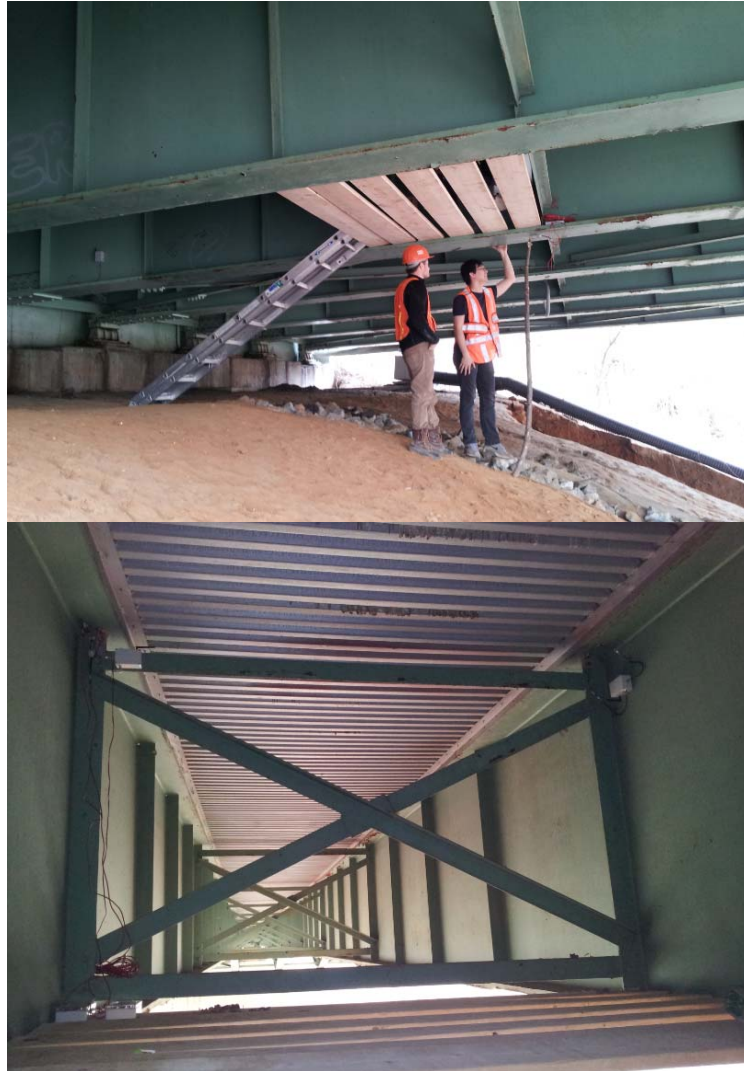
Figure 10 - Test Platform under the Bridge
