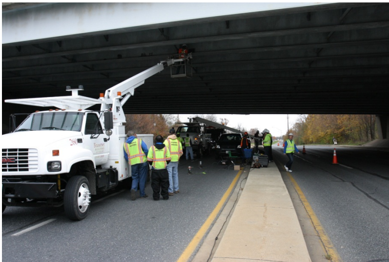
Figure 2. Field test on the I-270/Middlebrook Road Bridge, Maryland
