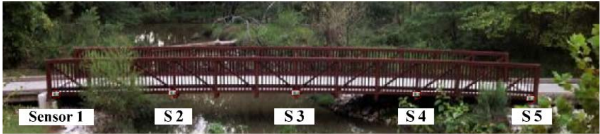
Fig. 2 Sensor locations on the test bridge
