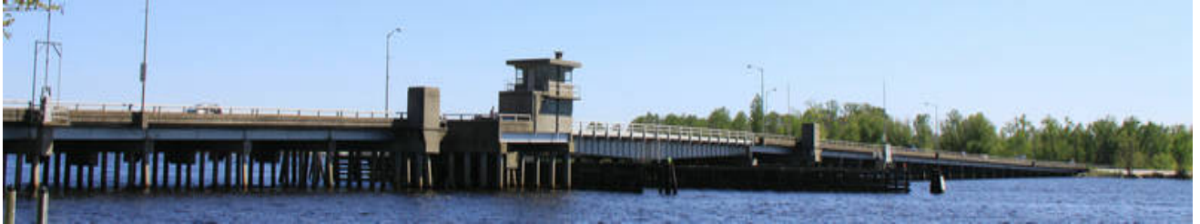
Figure 1 Full scope of the bridge
