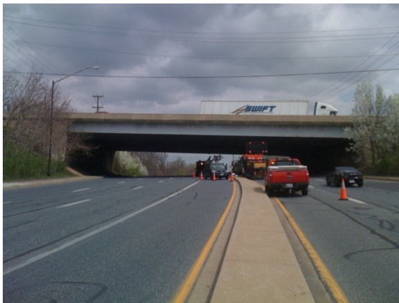
Figure 1. View of the bridge
